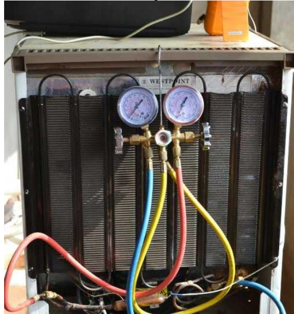
Figure 3: Shows the complete experimental set up of 60 litres domestic refrigerator. The ambient temperatures range from 17.0°C to 32.0 °C. The same procedure was carried out for R290 and R600a.
