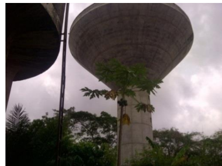
(a) 380 m 3 (100,000 gallon) reservoir (OAU) (b) Amina Way Elevated Reservoir at the UI
